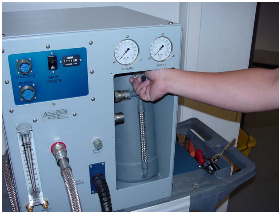
Figure 7-6. Remove compressor adsorber - Step 10
